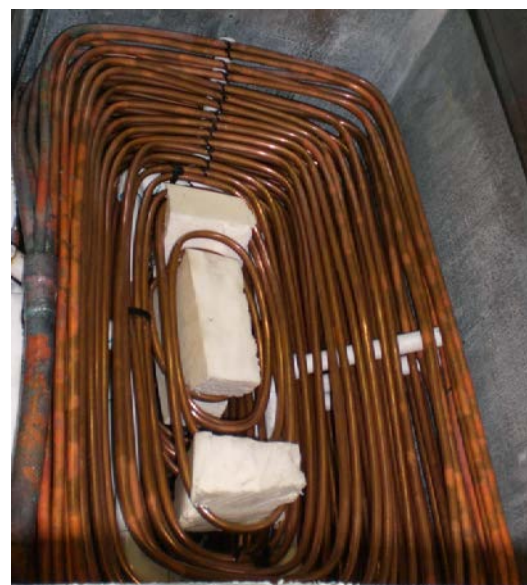
Figure 3: Example of condenser coil configuration to allow for adequate drainage of liquid refrigerant
