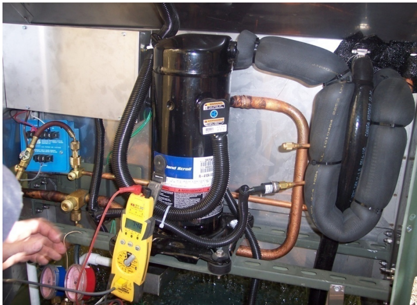
Figure 9: Gauges connected to operating evaporative condenser to verify correct charge
