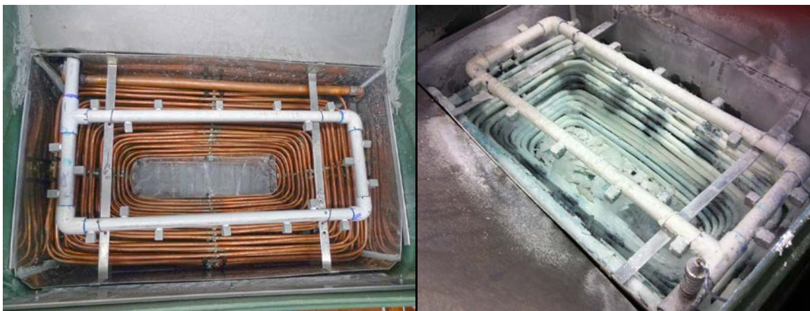
Figure 4: Condenser coil before (left) and after (right) prolonged operation without any water management strategies
