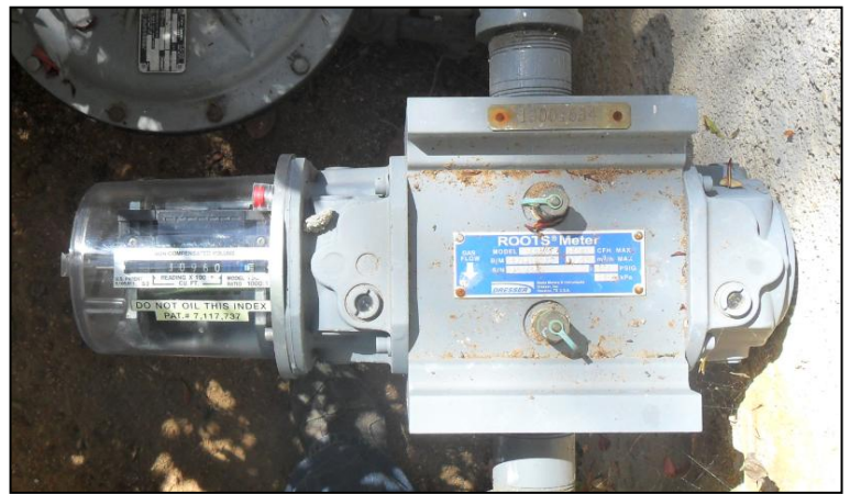
Figure 2.4: Typical Gas Meter—odometer (right)
