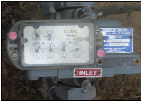
Figure 2.3: Typical Gas Meter—dial face (left)
